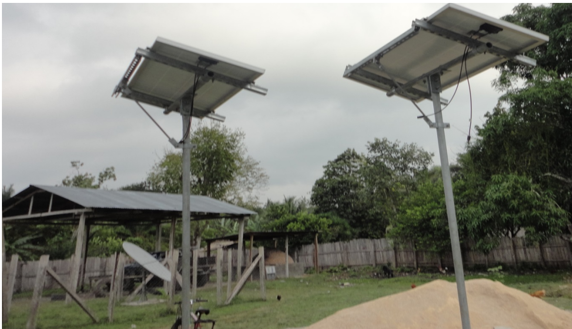
Solar panels installed by INDE in the village of Uaxactún / Photo: WCS
